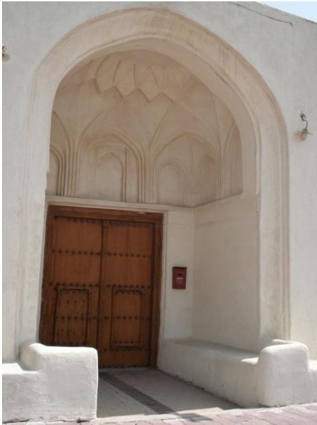
Figure 6: wooden door and use of white cement
