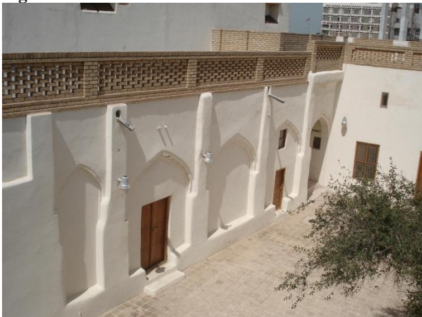
Figure 8: use of clay and white cement
